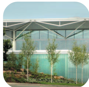
Existing terminal building
